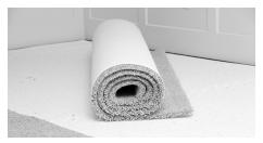
Underlay should be put on the floor first.
