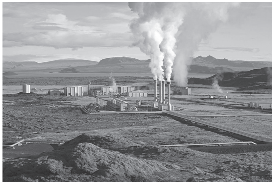
Geothermal power station
